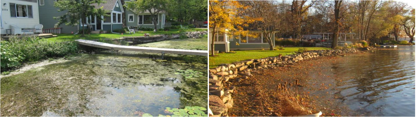
(Before and After pictures of the Breakwall project)
